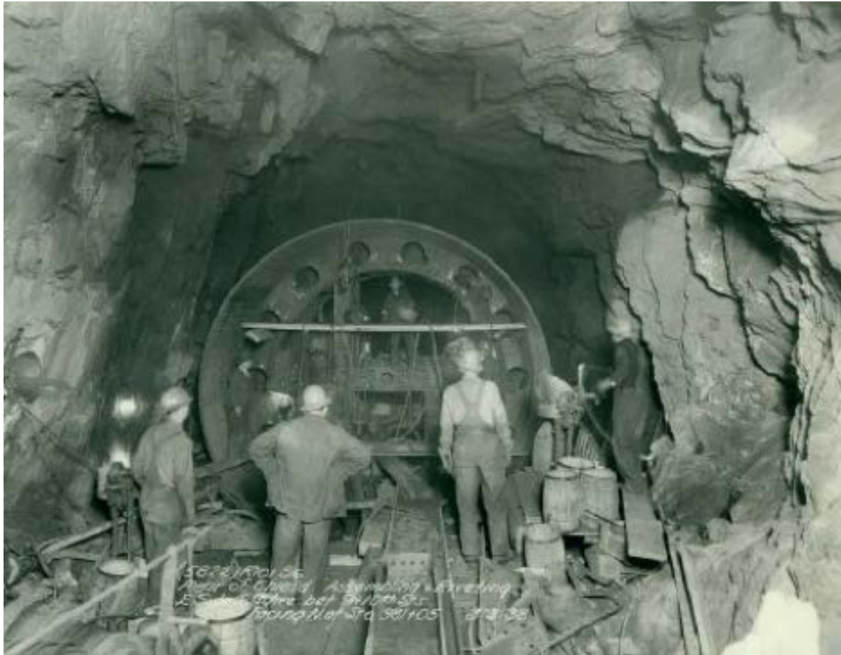
Laborers Doing Assembly and Riveting Work: Sixth Avenue Line (IND), 1938 New York Transit Museum Eugene Casey Tunneling Collection
