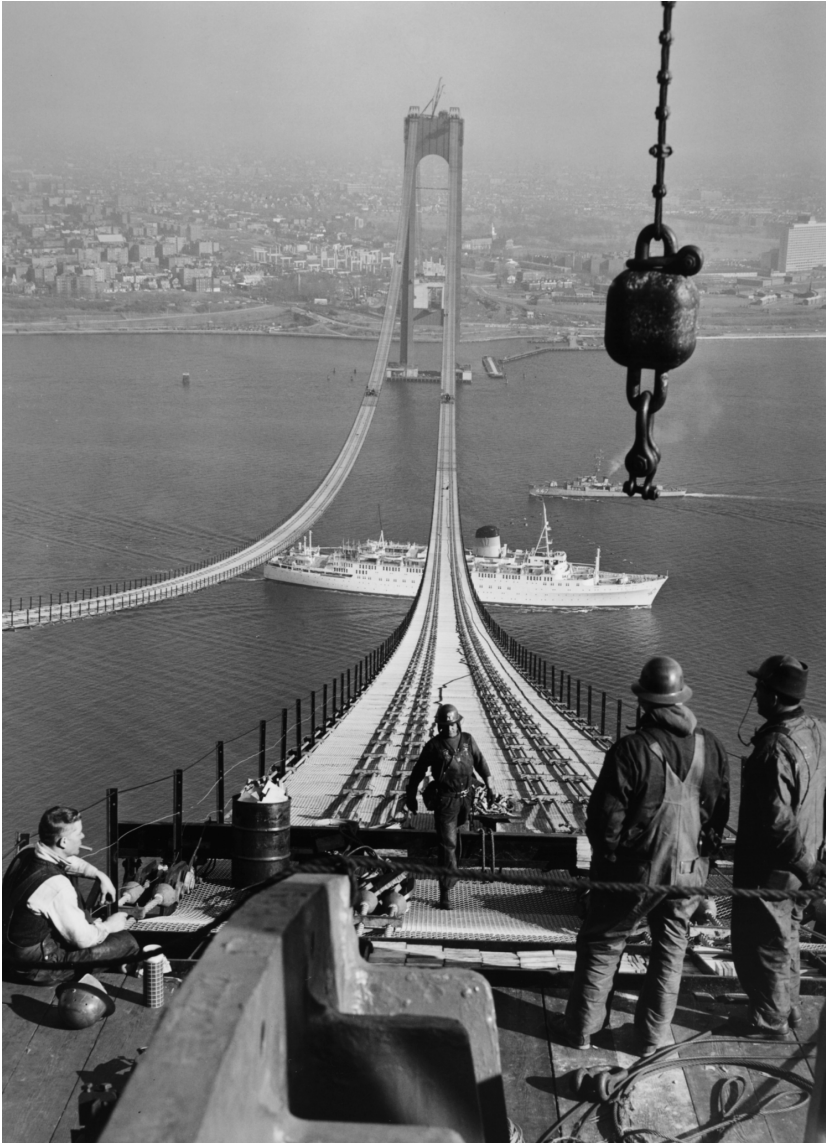
Verrazano-Narrows Bridge catwalk, featured in Spanning the Narrows .
